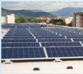
Flat Roof Installation
